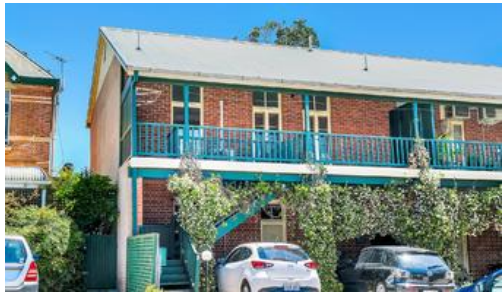
Unit 4, 422 Carrington Street, Adelaide
