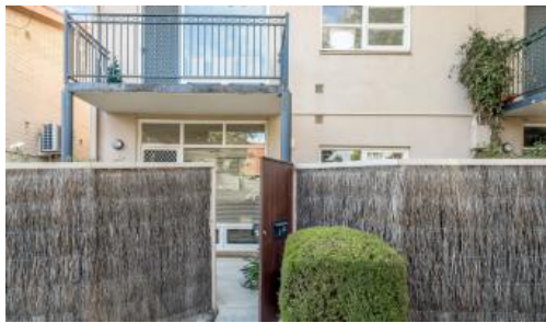
Unit 1/ 1A Stannington Ave, Heathpool
