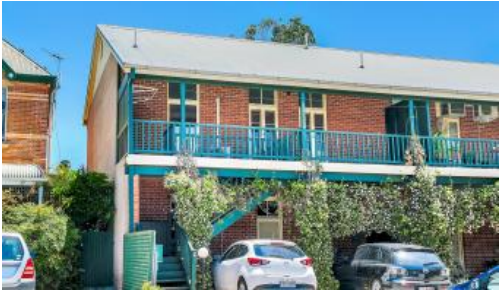
Unit 4, 422 Carrington Street, Adelaide
